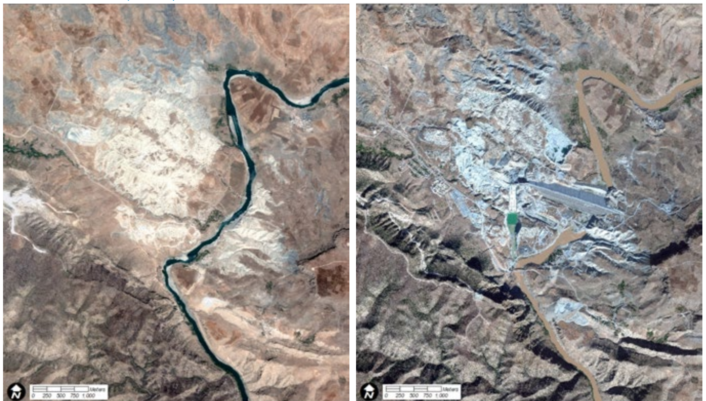
FIGURE 2: EVOLUTION OF ILISU DAM CONSTRUCTION BETWEEN JANUARY 2009 (LEFT) AND NOVEMBER 2016 (RIGHT)
